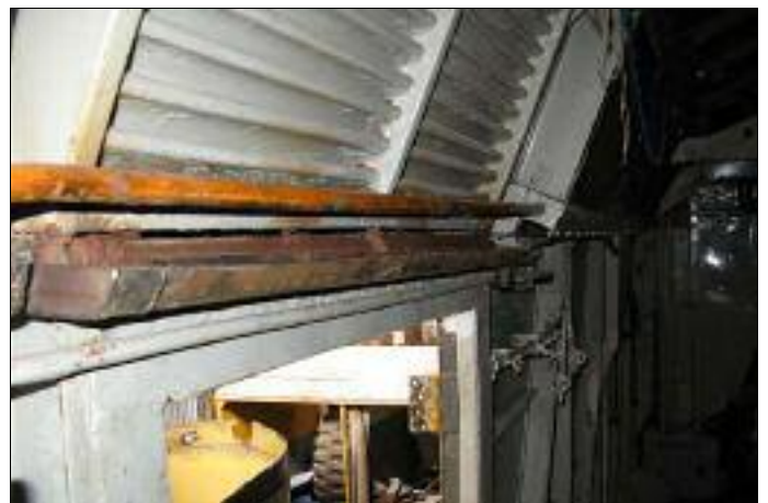
New internal gutters welded in place.
